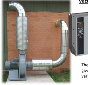
The combination of a direct drive vacuum unit and a frequency inverter with PID regulation enables us to make a constant suction pressure level and a vacuum unit with no maintenance at all.
