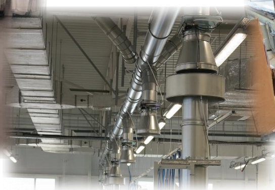
Automatic pipe connection for movable cutters
